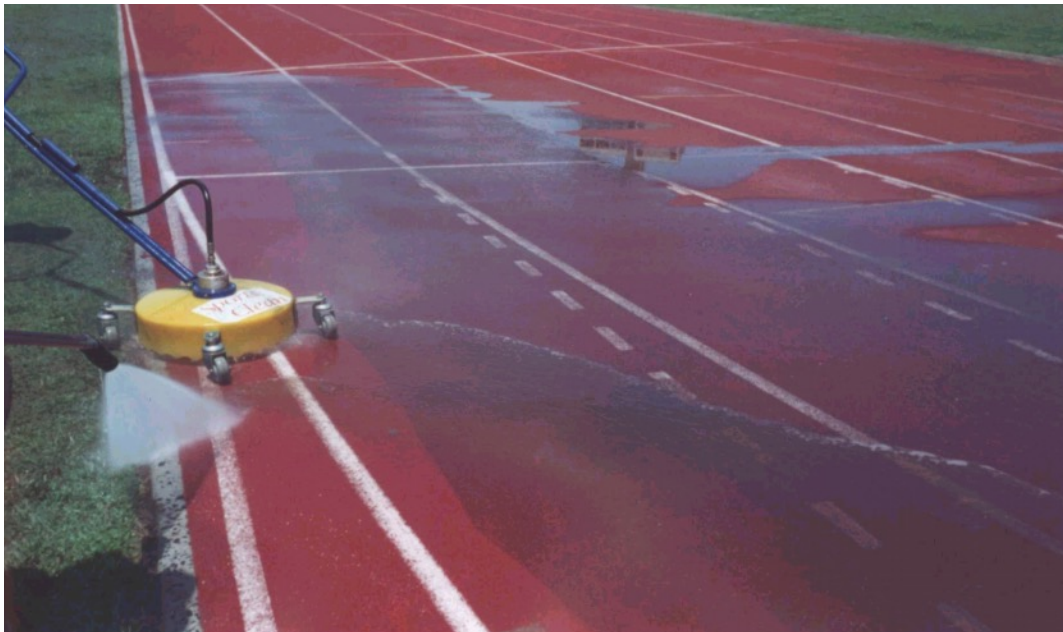
Washing of track to be done with rotary cleaning head & hand held pressure cleaner
